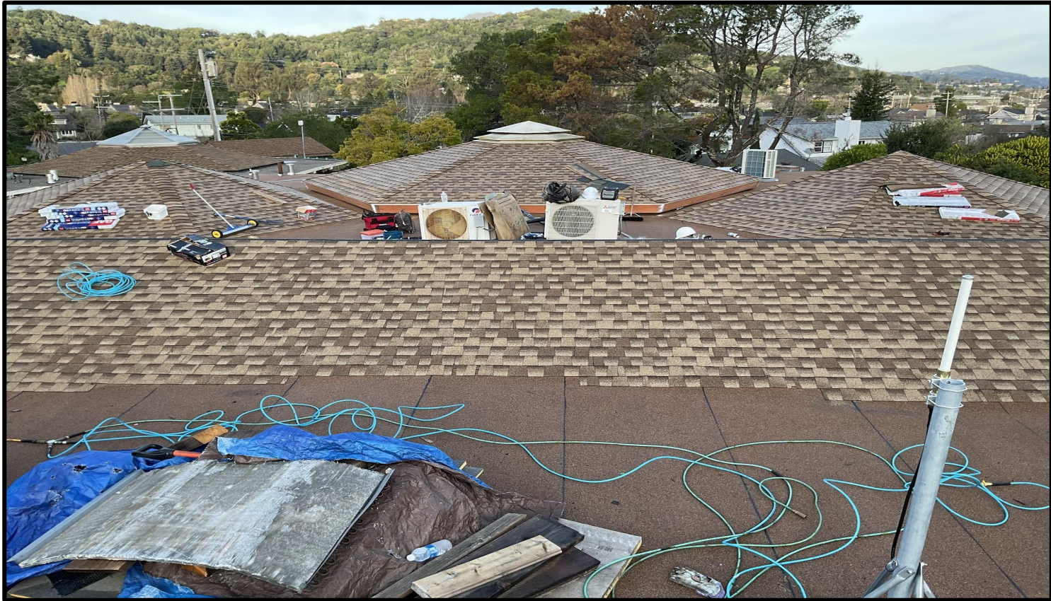
GRANADA PROPERTY - Roofing Work on the Omega Building
