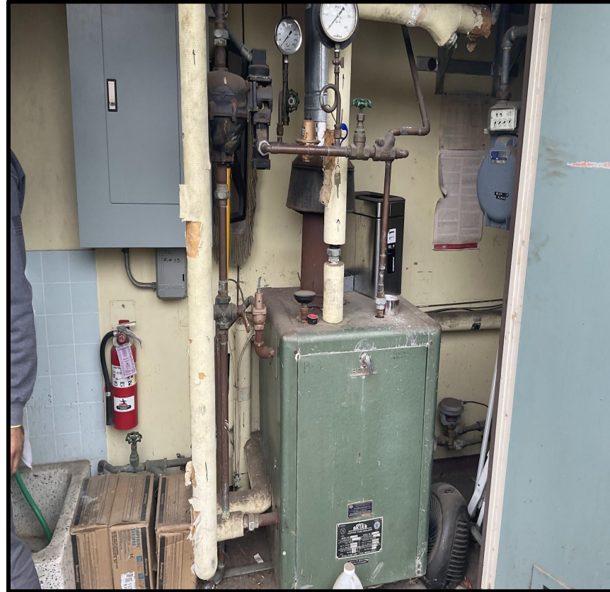
GRANADA PROPERTY - Boiler Removal
