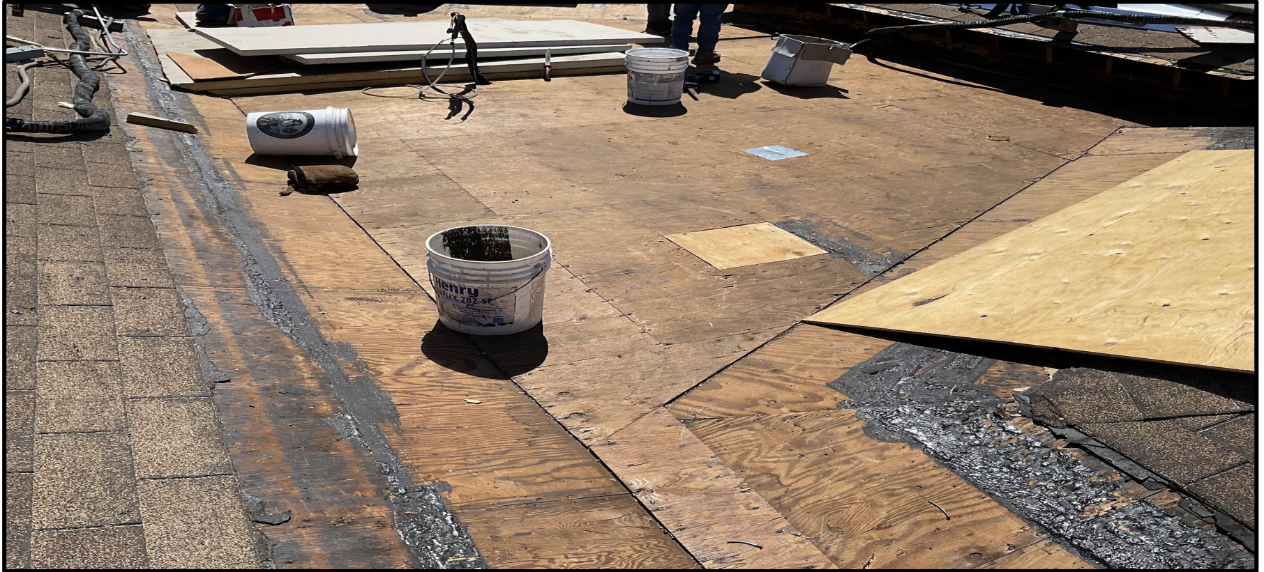
GRANADA PROPERTY - Roofing Work on the Omega Building
