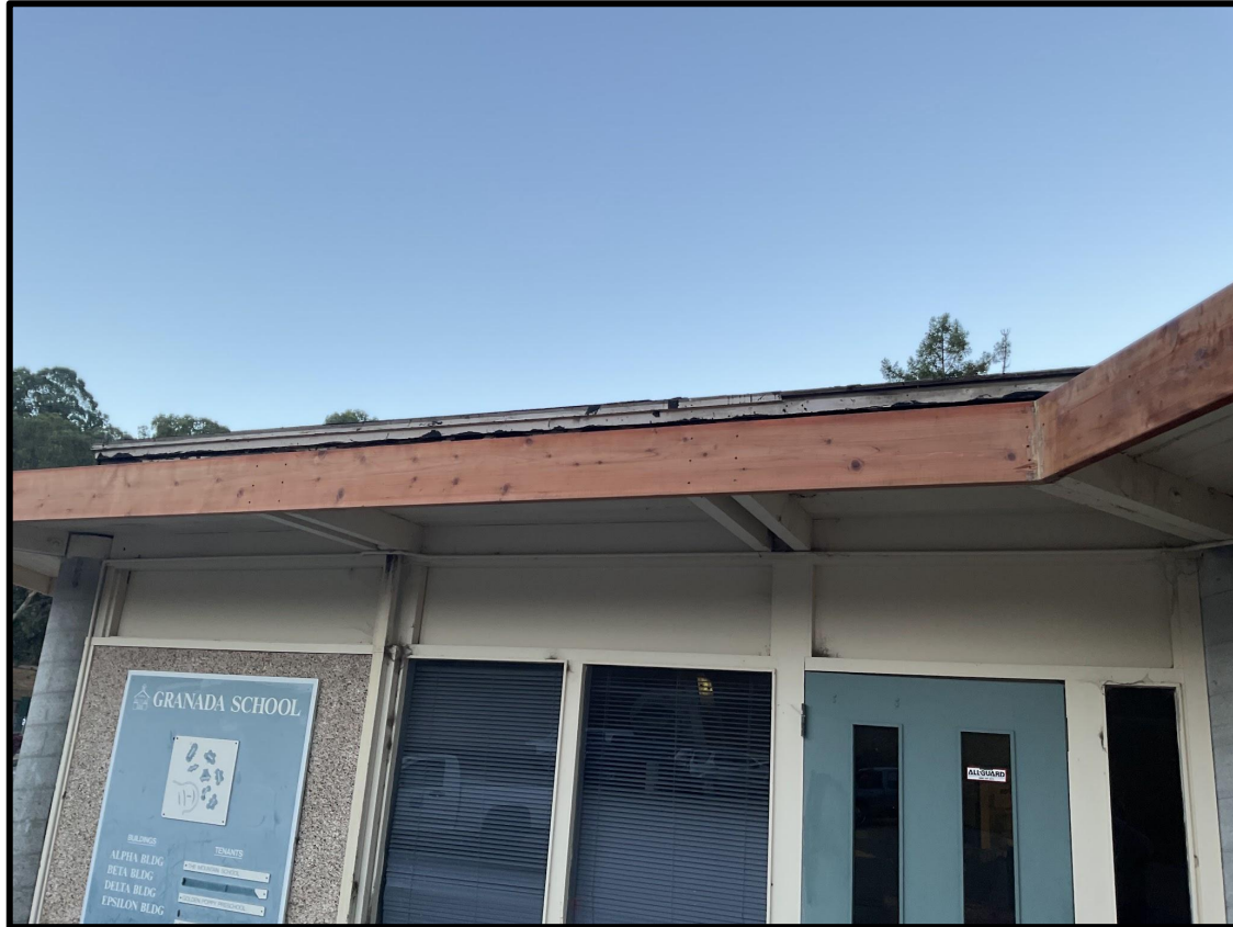
GRANADA PROPERTY - Roofing Work on the Omega Building
