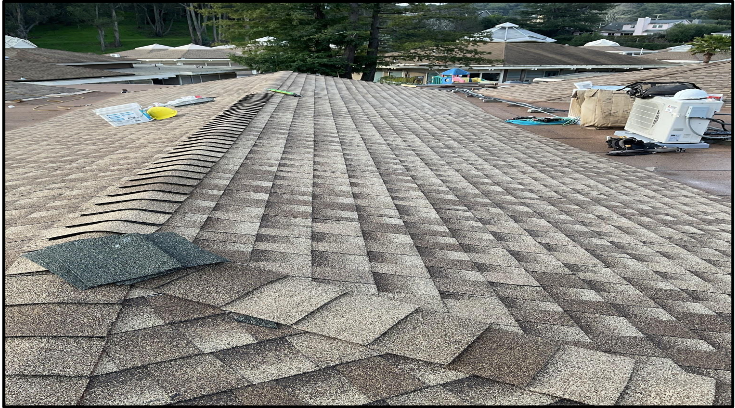
GRANADA PROPERTY - Roofing Work on the Omega Building
