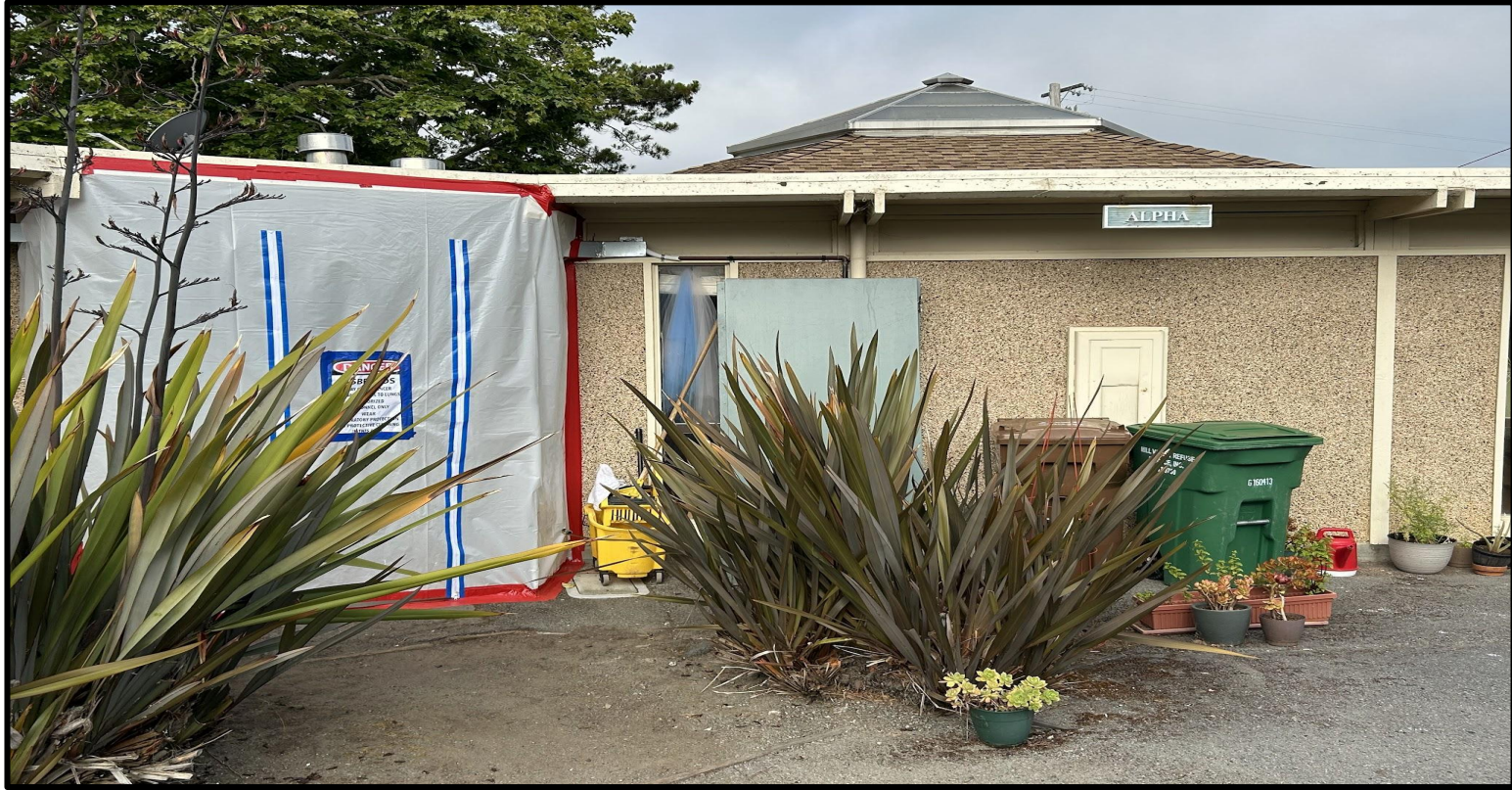
GRANADA PROPERTY - Asbestos Removal
