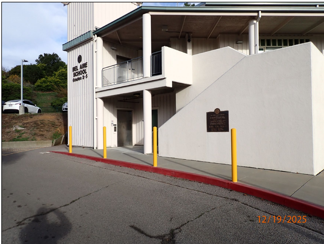
Item 7 – Elevators have been installed to provide access to 2 nd story structures.
