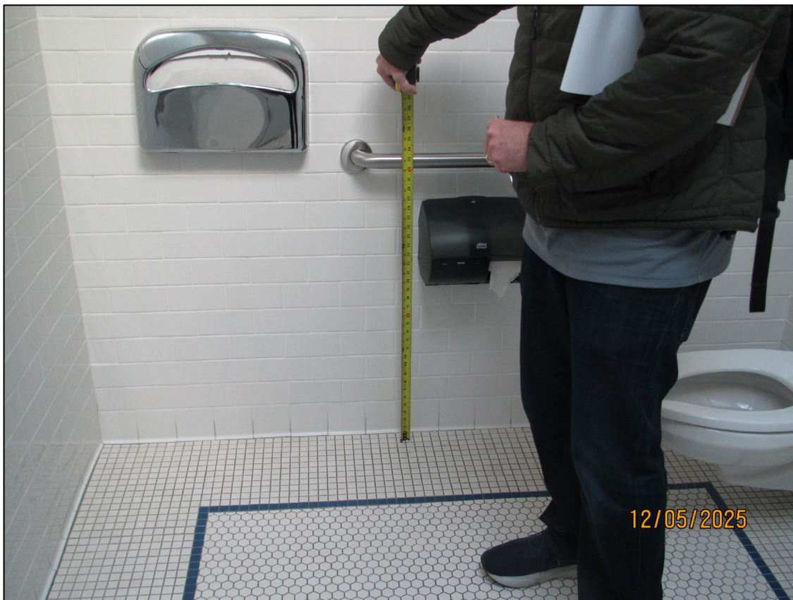
Item 12 – Grab bars have been installed at all bathrooms.
