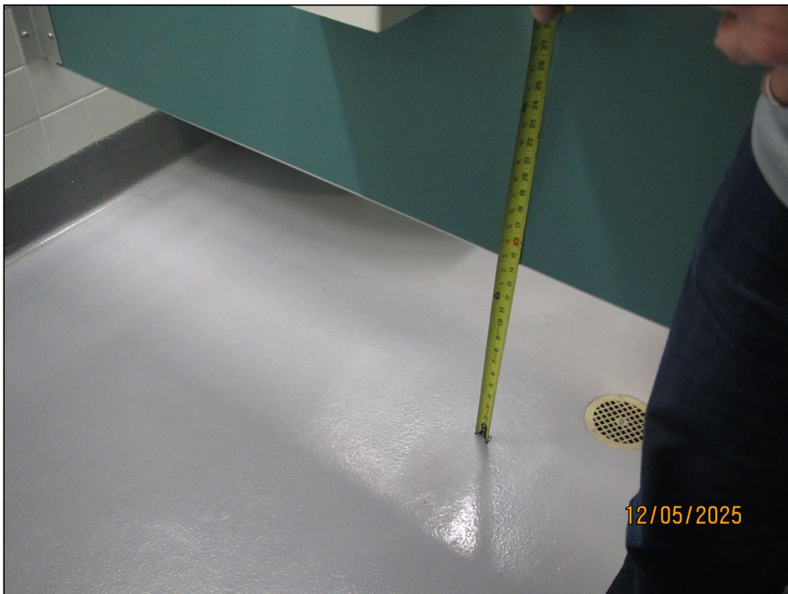
Item 16 – Partitions offer proper clearance for wheelchair turn around.
