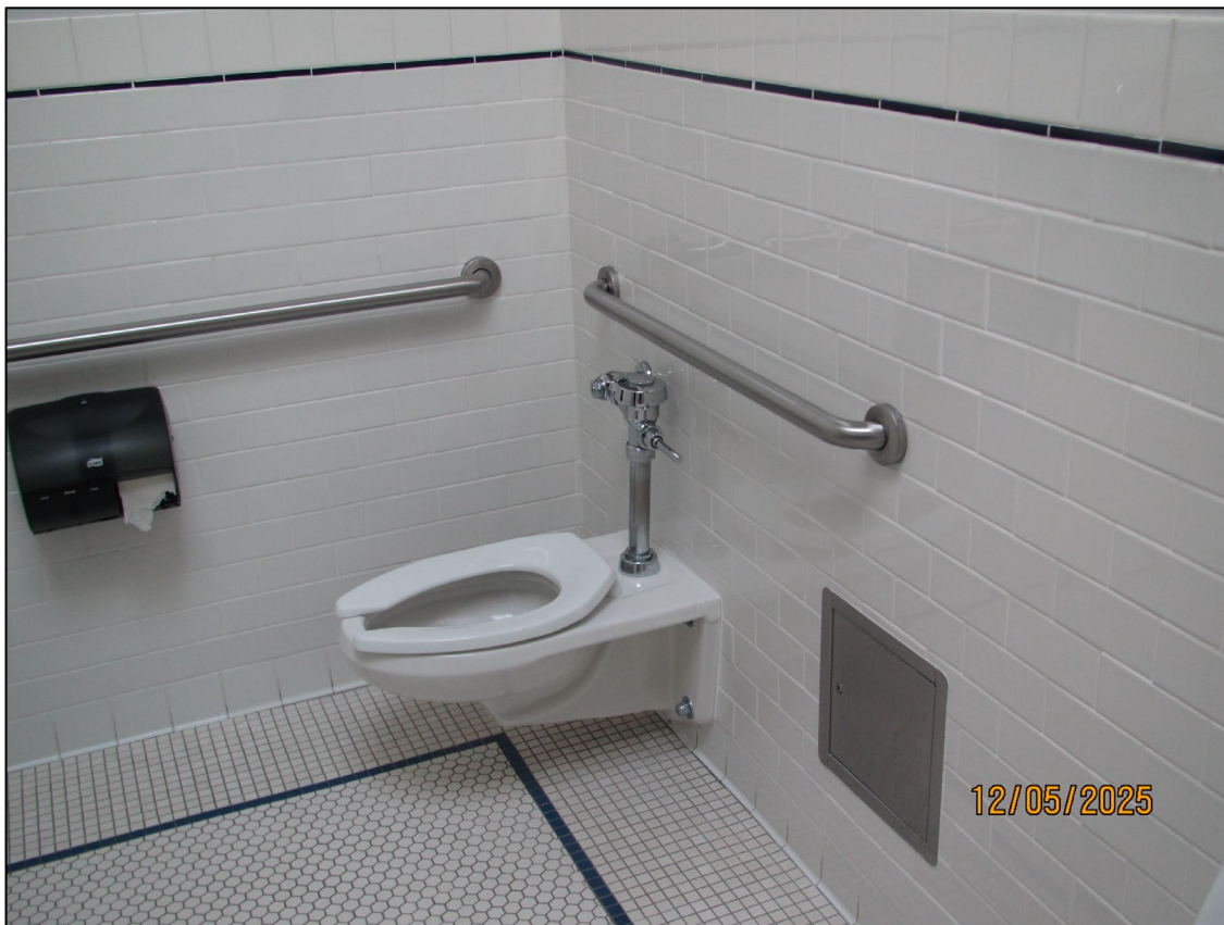
Item 14 – Flush valves located on open side of the water closet.
