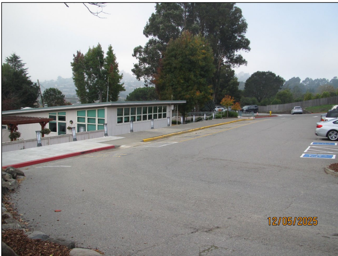
Item 2 – Loading area used for student drop off.
