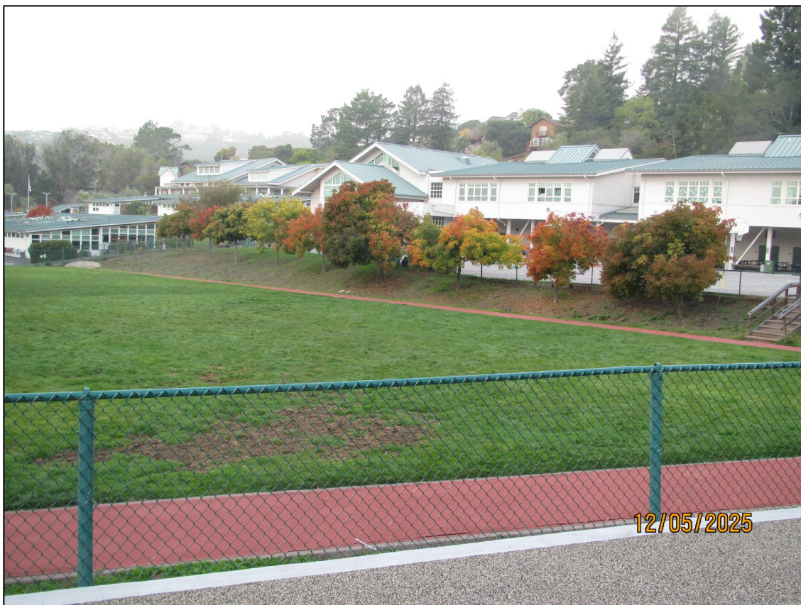
Item 10 – An accessible route to the field was difficult to identify.
